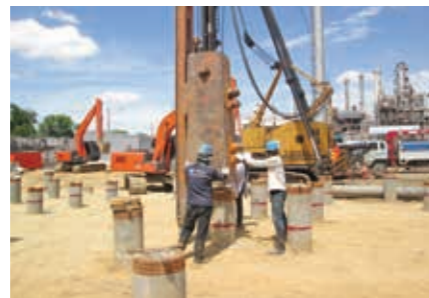
Concrete piling works
