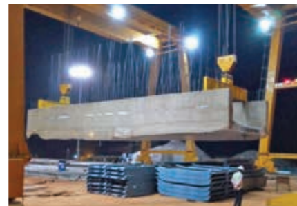
Underside of the bridges & piers etc
