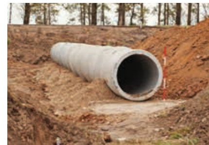
RCC pipes for use in underground where sulphate concentration is high
